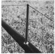
**6.** Using a piece of wood, plastic or well rounded metal (not a screwdriver!) push the wire all the way down into the plastic end-cap. It should "snap" into place. If for any reason it does not and stays loose, tape over the end of the plastic so that the wire cannot fall out when it goes slack.
